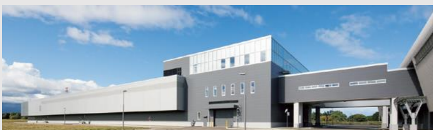
Ishikari Data Center Building 3, built by SAKURA Internet Inc. in Ishikari City in December 2016
